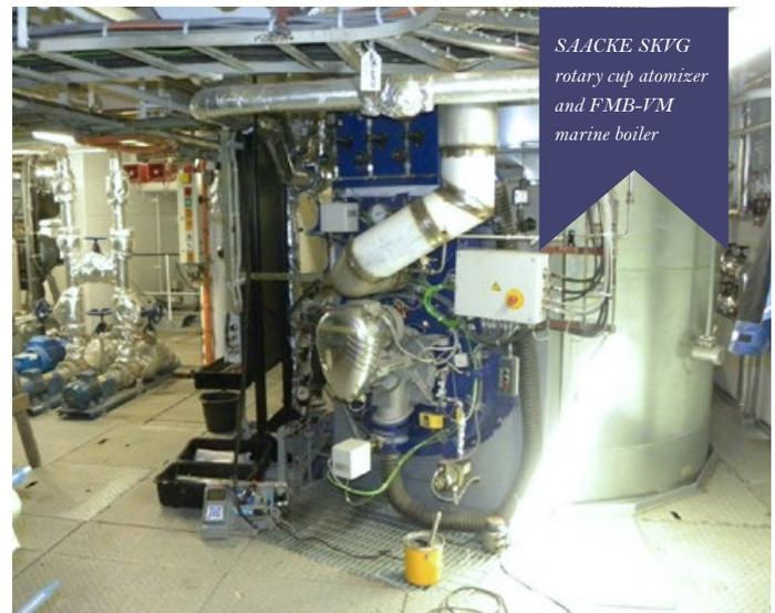
SAACKE SKVG rotary cup atomizer and FMB-VM marine boiler
