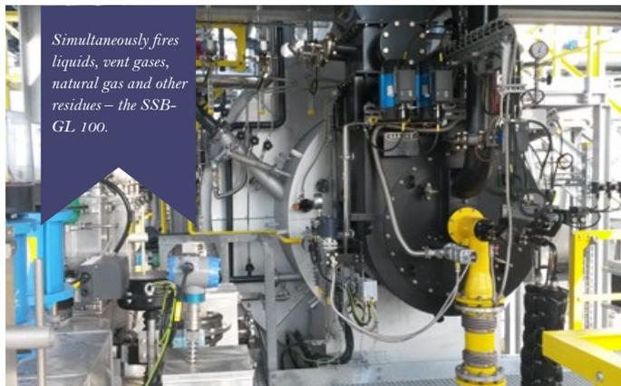
*Simultaneously fires liquids, vent gases, natural gas and other residues – the SSB-GL 100.*
