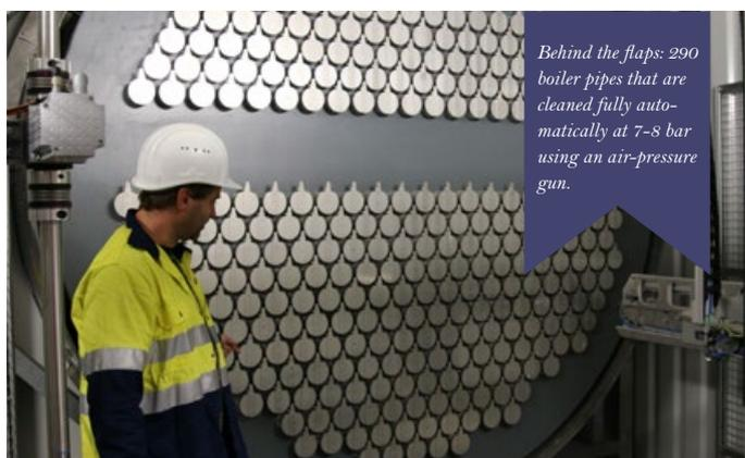
*Behind the flaps: 290 boiler pipes that are cleaned fully automatically at 7-8 bar using an air-pressure gun.*
